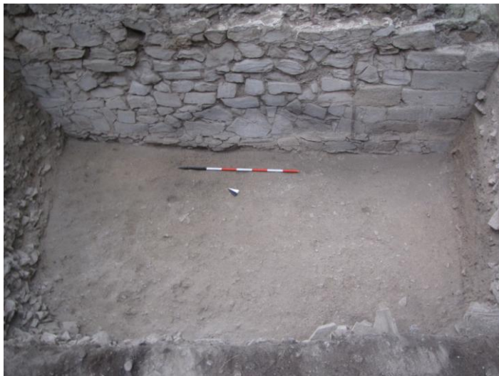
Fig. 5. Southwest corner of the perimeter wall.
